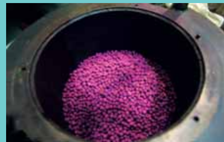
▲ Brightly colored Purafill pellets filter out odors in the chambers. The deeper the chamber goes, the more intense odors become.
